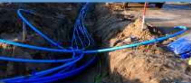
Cable- and Pipelines
