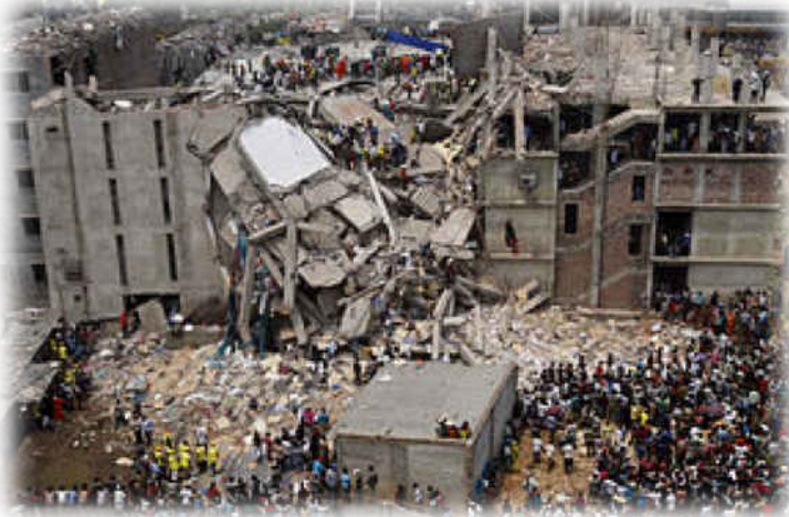
Rana Plaza, Bangladesh, collapsed in 2013 (killed 1,129)
