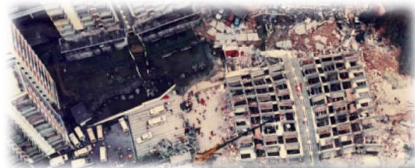
Highland Tower collapsed in 1993, Ulu Klang, Selangor, 48 killed
