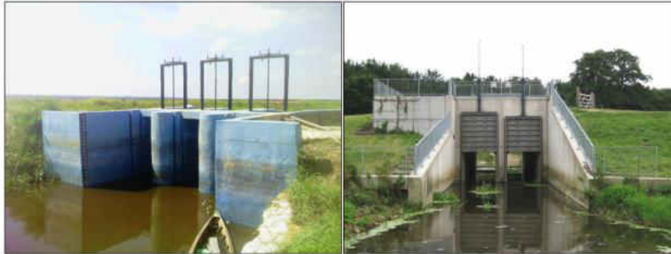
Sluice gates – Manually operated or by motor
