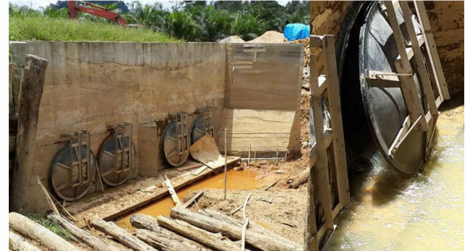
Flap gates – Will close automatically if the water level outside the embankment is higher
