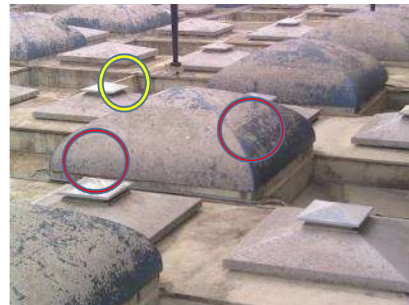
cold spots (red) are indication of trapped moisture, whilst the hot spot (yellow) are signs of delamination or subsurface void.
