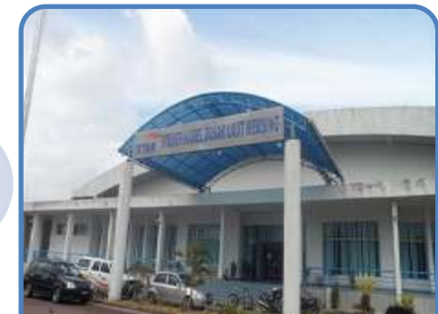
Cable Landing Station
