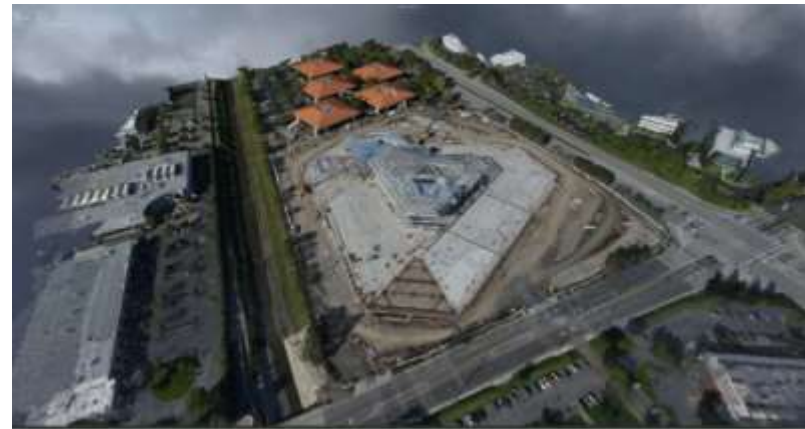
Point cloud of a construction site, viewed in a VR environment
