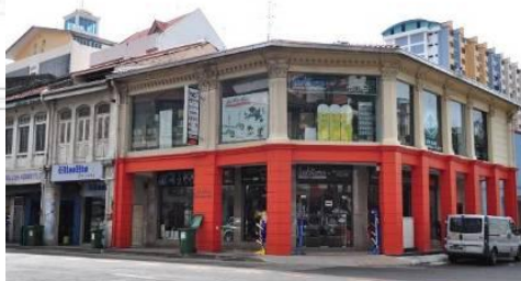
Shop houses - above tunnel alignment
