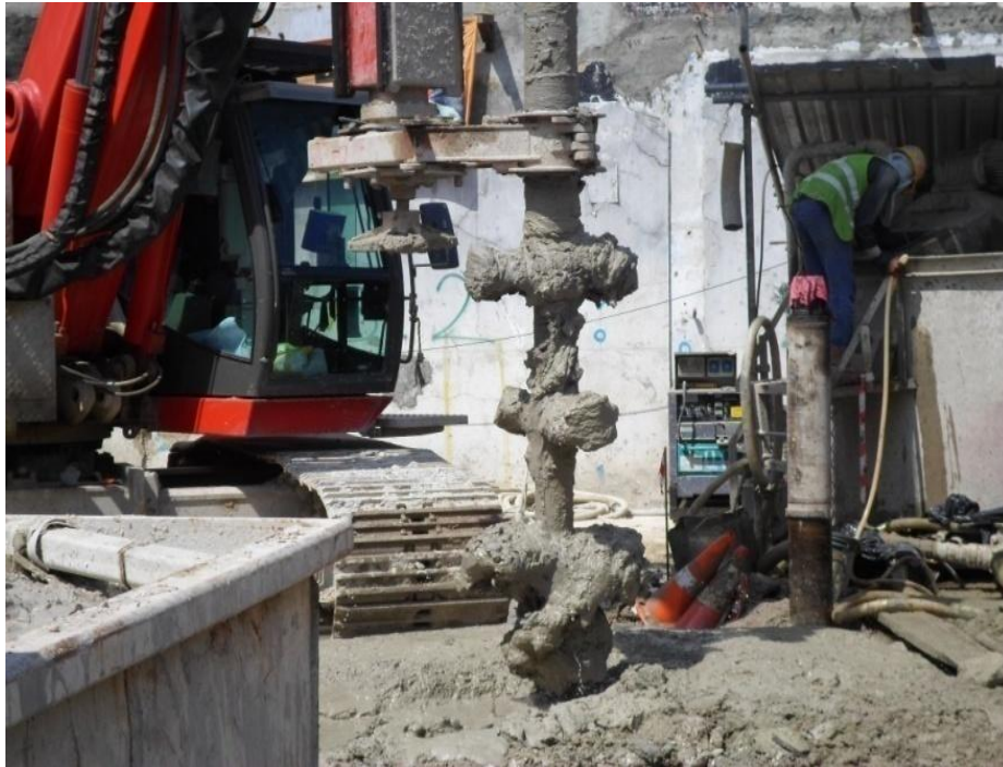
Installation of WSM in progress
