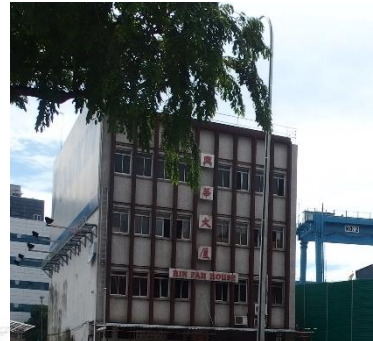
Hin Fah House - adjacent to station
