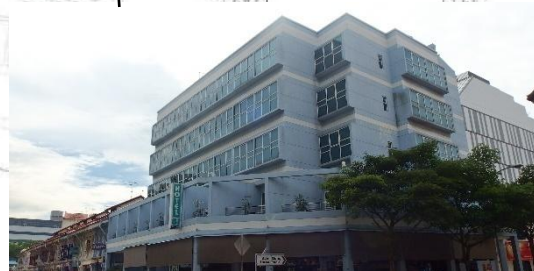
Hotel 81 - above tunnel alignment
