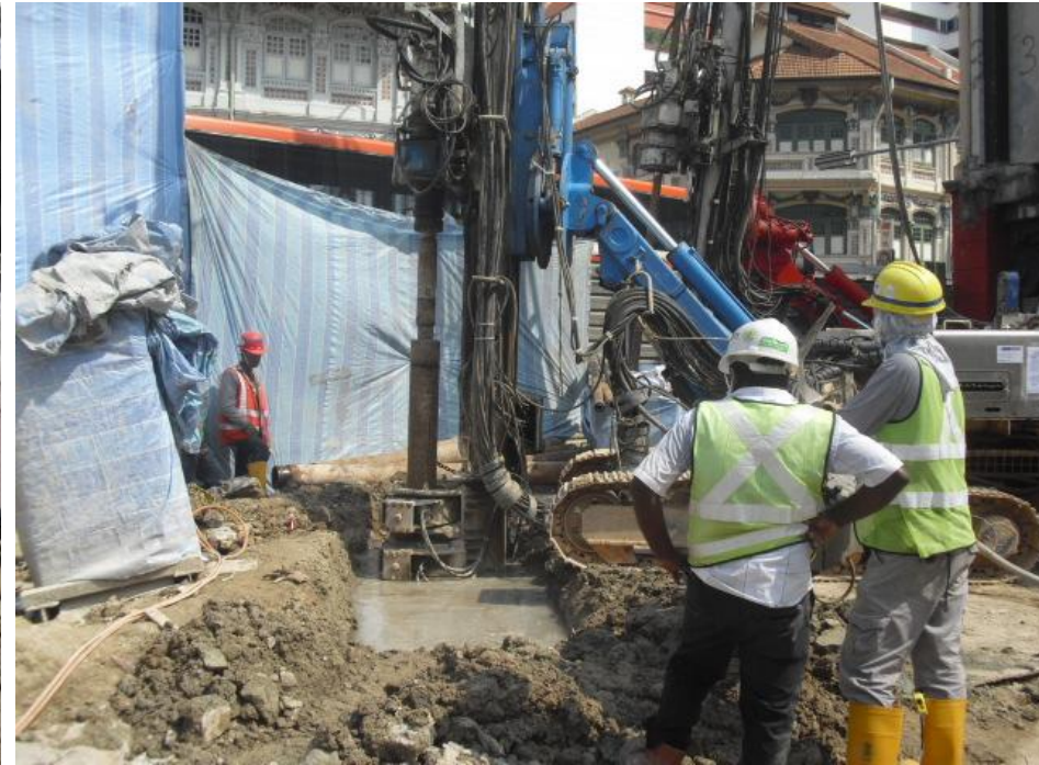
Installation of JGP in progress
