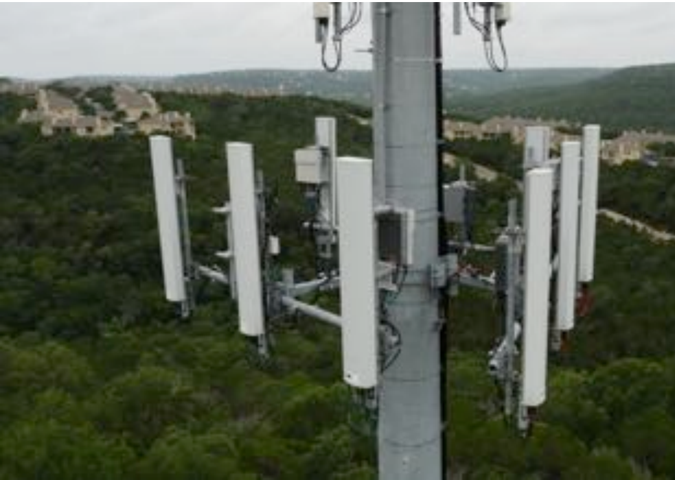
Example: Telco Tower Inspection
