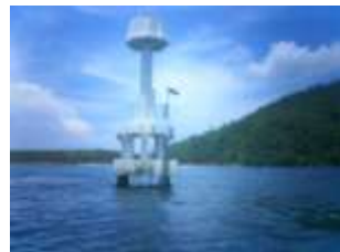
Tide Gauge Station
